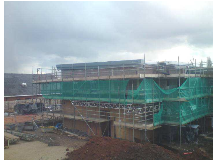
Render Prep Work To Gable Elevation
