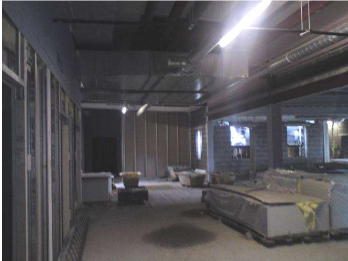
1 st Fix M&E To First Floor
