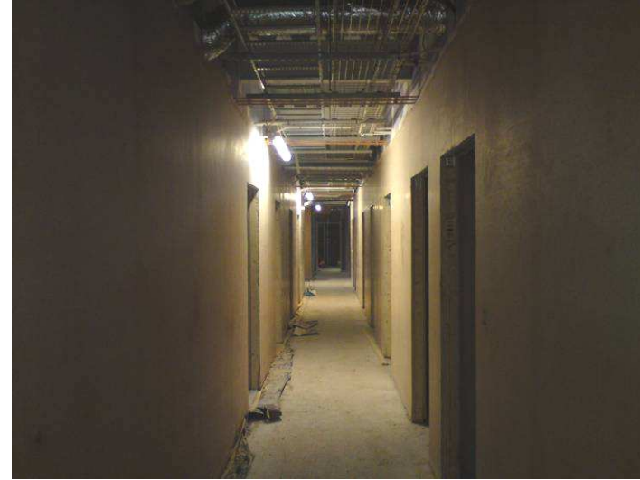
Plaster Skim To Ground Floor
