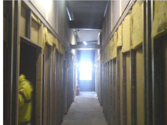
1st Floor Partitions Ready For Back Boarding
