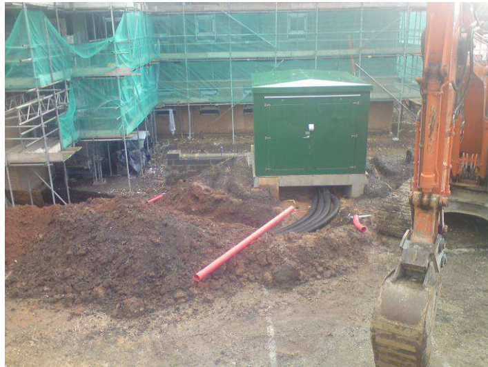
Incoming Electric Ductwork to Substation
