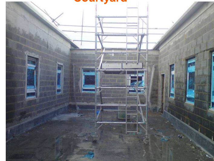
Render Prep Work To Internal Courtyard
