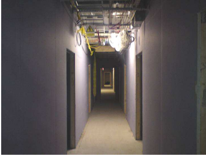
2 nd Fix Partitions To Ground Floor
