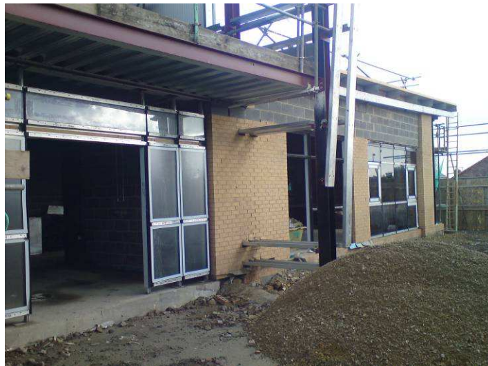
Glazing To Front Entrance
