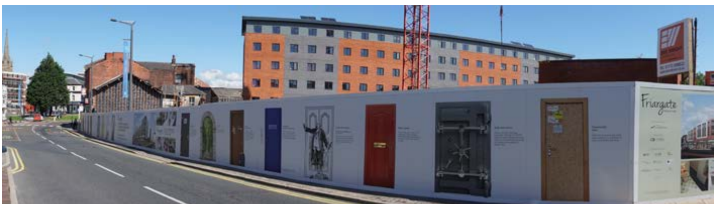
New hoarding has been erected around the site at Friargate
